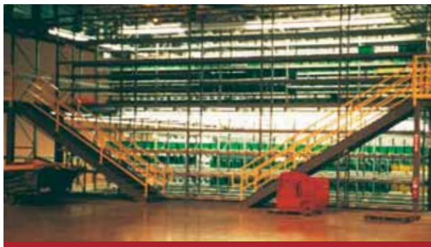
Multi-level Wide Span Pick Module
